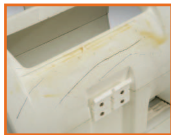
Crack and chip repair, repaint
